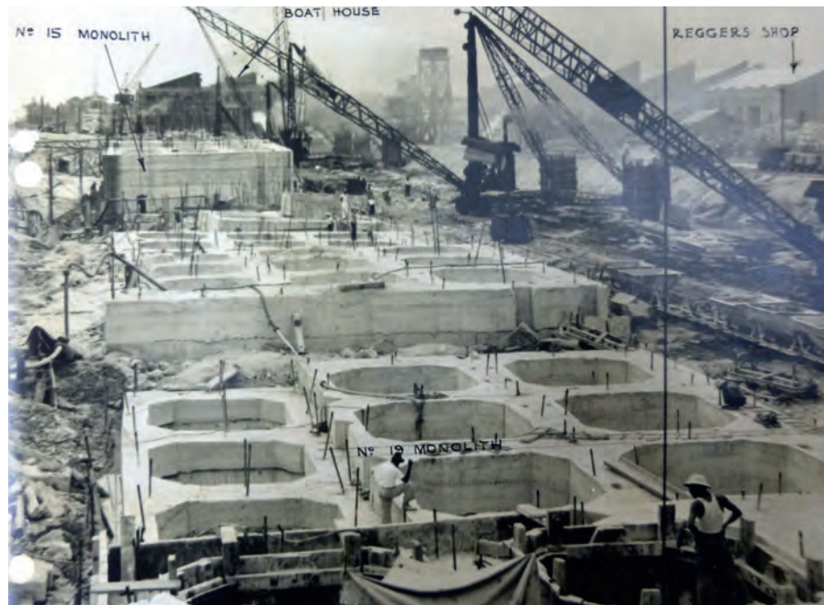
North Wall looking east showing monoliths in various stages of construction. The building in the background with serrated roof edge is the Boat House at the mid-point of the North Wall, 11 October 1940. (Photo: TNA ADM195/118-A460.)
