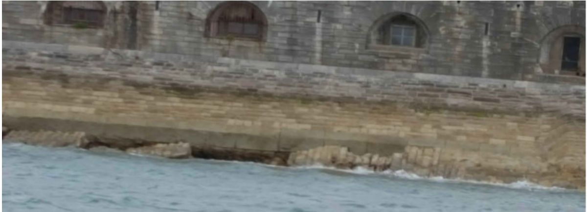
Figure 37 6 Aug 2019. Damage to sea wall in front of Blockhouse main battery. CHD.
