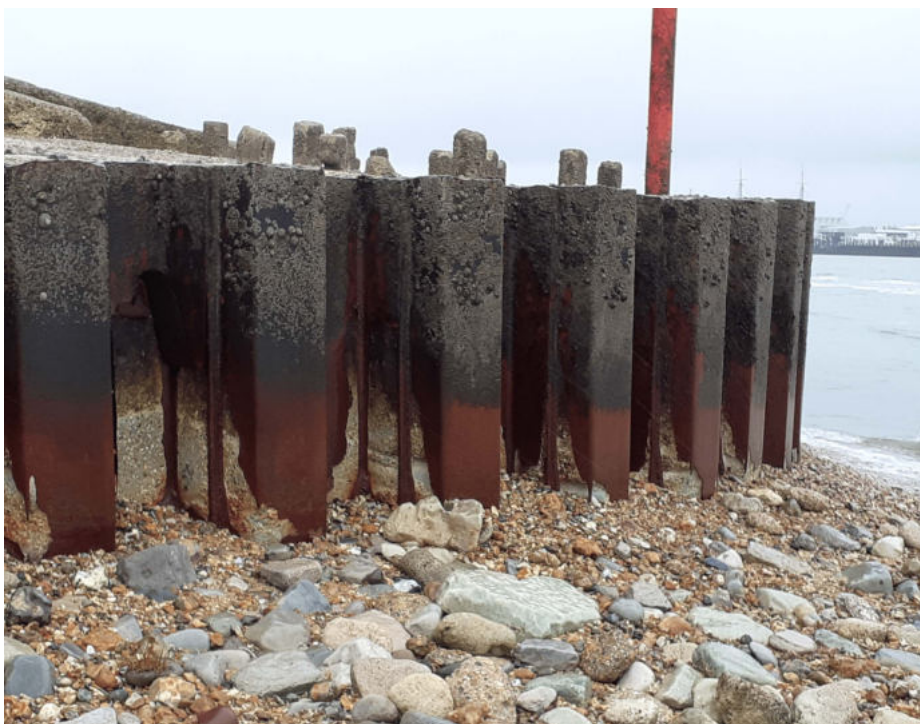
Figure 40 2020. The harbour entrance piles, looking North. The steel is shot and the concrete backing, seen through the piles, does not look in good shape. AM.
