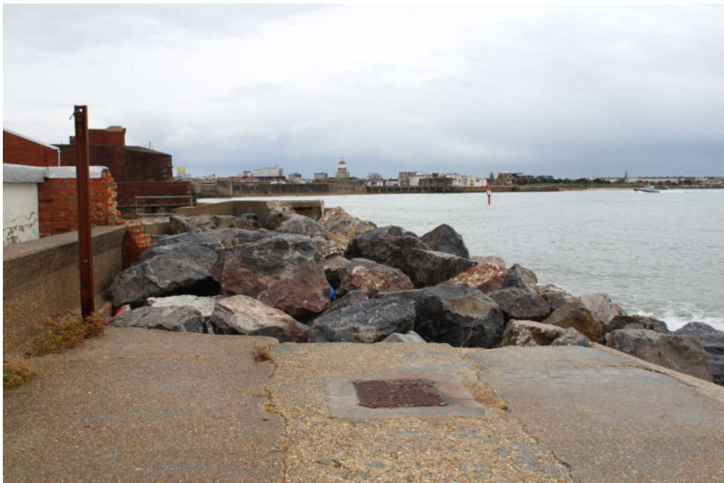
Figure 31 14 Jan 2014. The repair looks suitably impressive but, in practice, probably served to expedite the erosion process. CHD.
