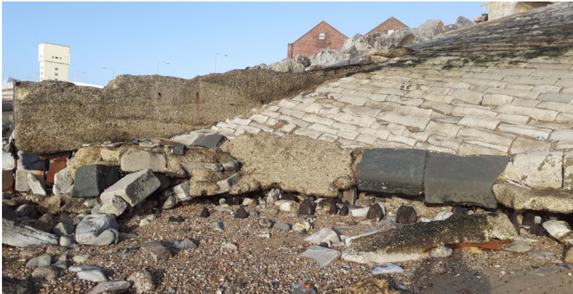
Figure 43 2020. A graphic illustration of the undermining process. Once the water gets under the existing defences, the only ‘resistance’ here is sand and shingle. AM.
