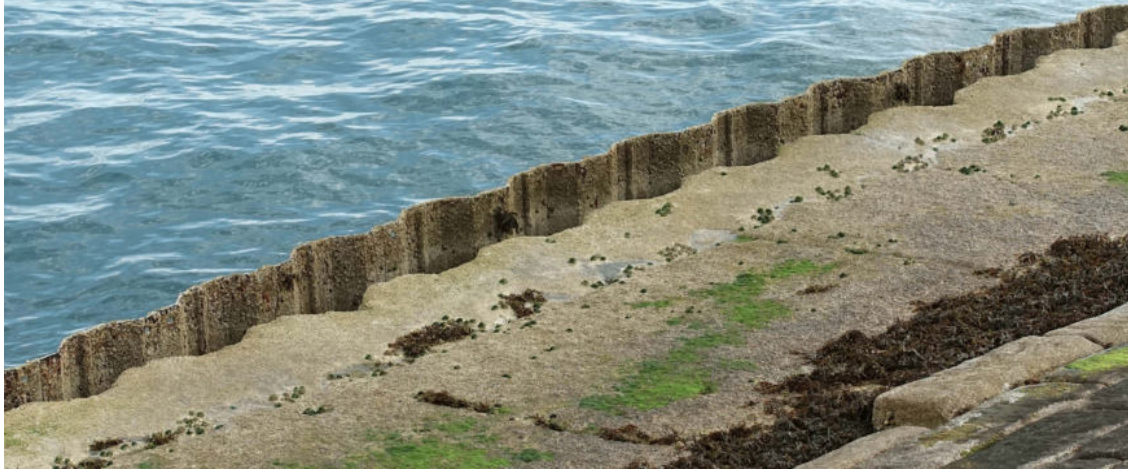
Figure 51 Aug 2020 Pile damage opposite the old submarine school. CHD.
