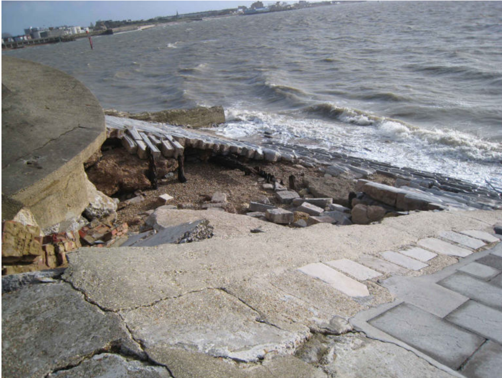
Figure 30 6 Jan 2014. The explosive nature of the event is self-evident; most of the stone facings have been blown clean out of the hole. CHD.
