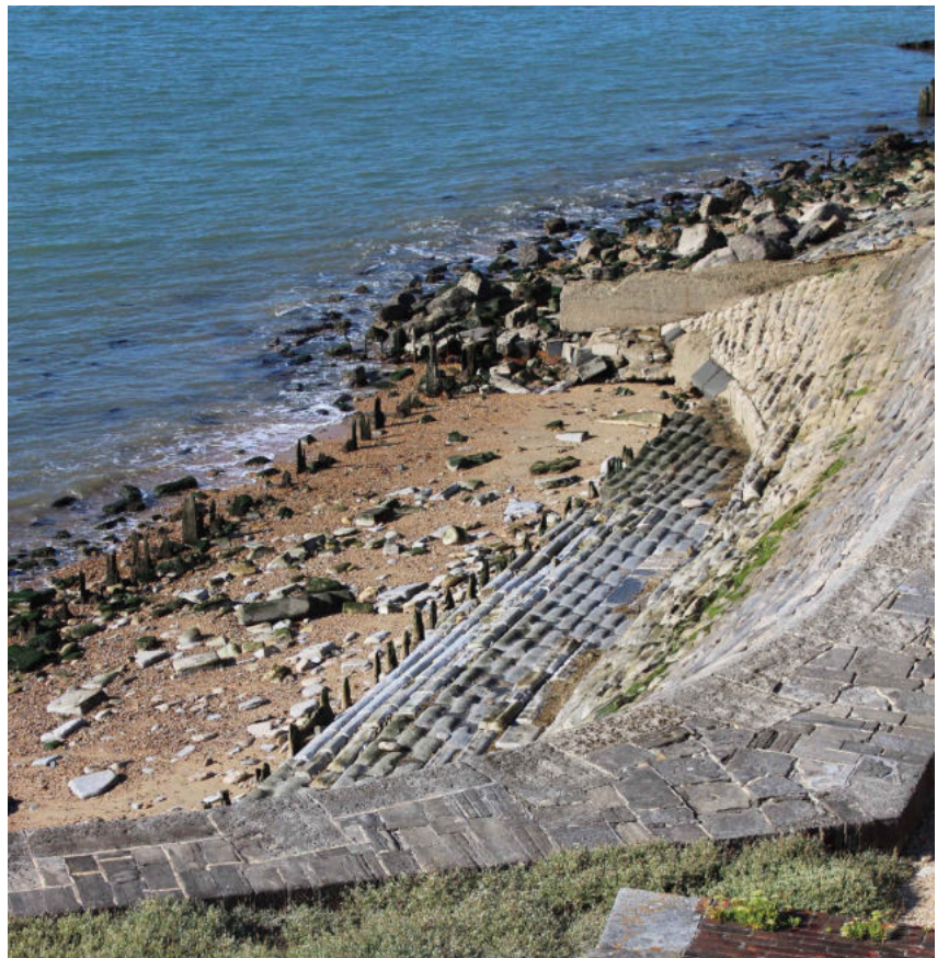
Figure 45 August 2019. The same position as above. The 1900s piles are almost gone. CHD.
