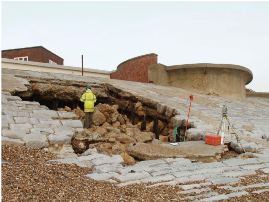
Figure 28 2006. The hole in the wall, in almost the same spot. Note the WW11 construction to the right; [source unidentified].
