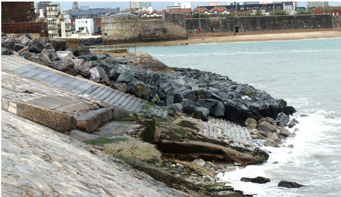
Figure 49 The repair stops short of the sheet piling, apparently due to some issue with the MMO licence extension. CHD.
