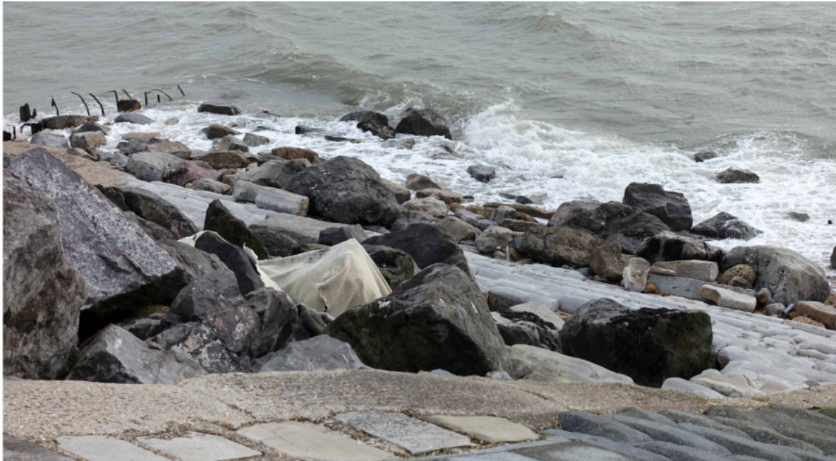
Figure 47 Feb 2020. The 2014 ‘temporary emergency repair’ after Storm Dennis; note how the rock armour has been tossed around like marbles; the repair was failing; CHD.
