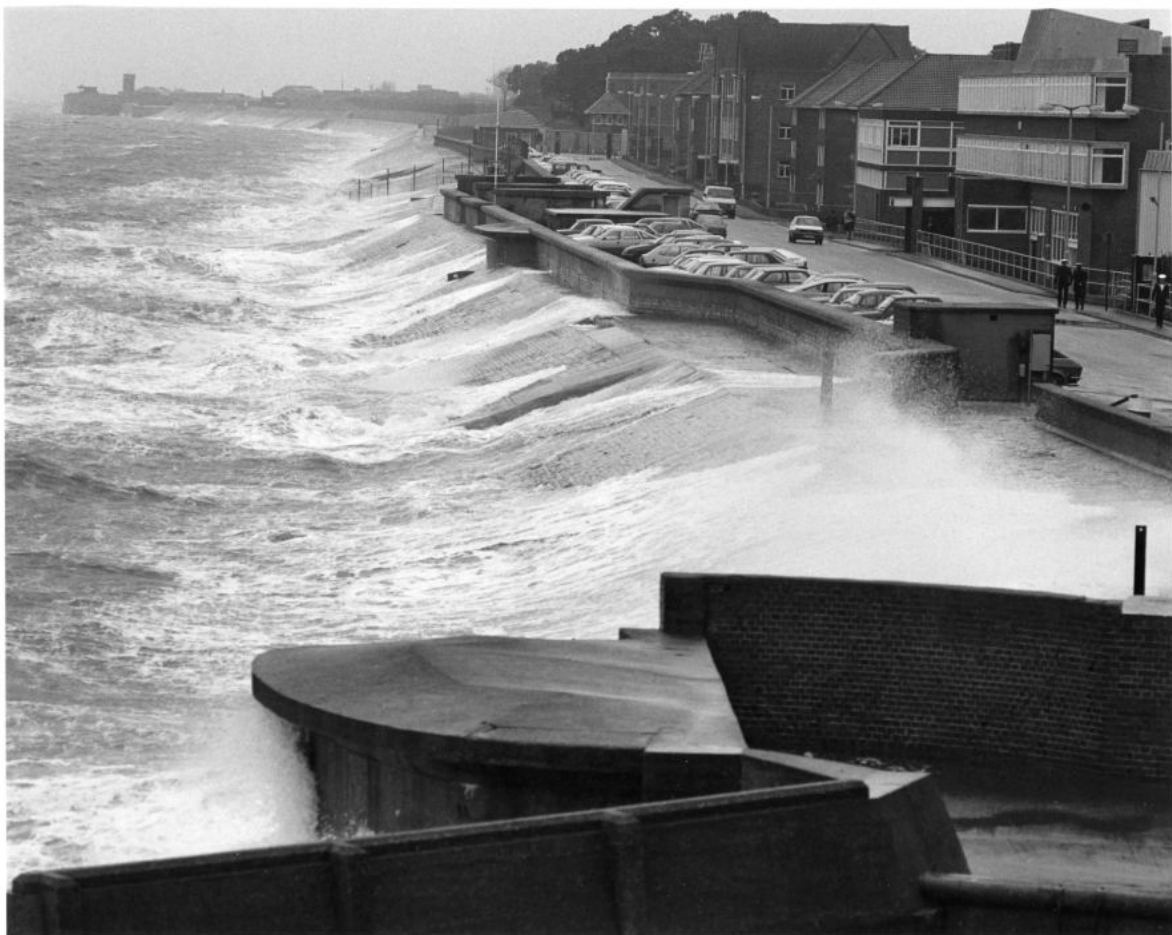
Figure 52 1987. The scene during a moderate gale, looking from the Fort towards Haslar. Potential building site to the right. In a storm, the wall takes a terrible battering. A description of one such event reads, 'large volumes of seawater pass over the sea wall carrying with it quantities of shingle and large concrete slabs. The road became impassable ...'. As noted earlier, the large concrete structure in the foreground was carried away in Dec 2013. The subsequent temporary emergency work, never replaced with a permanent repair, was itself badly damaged by Storm Dennis in Feb 2020. MoD.
