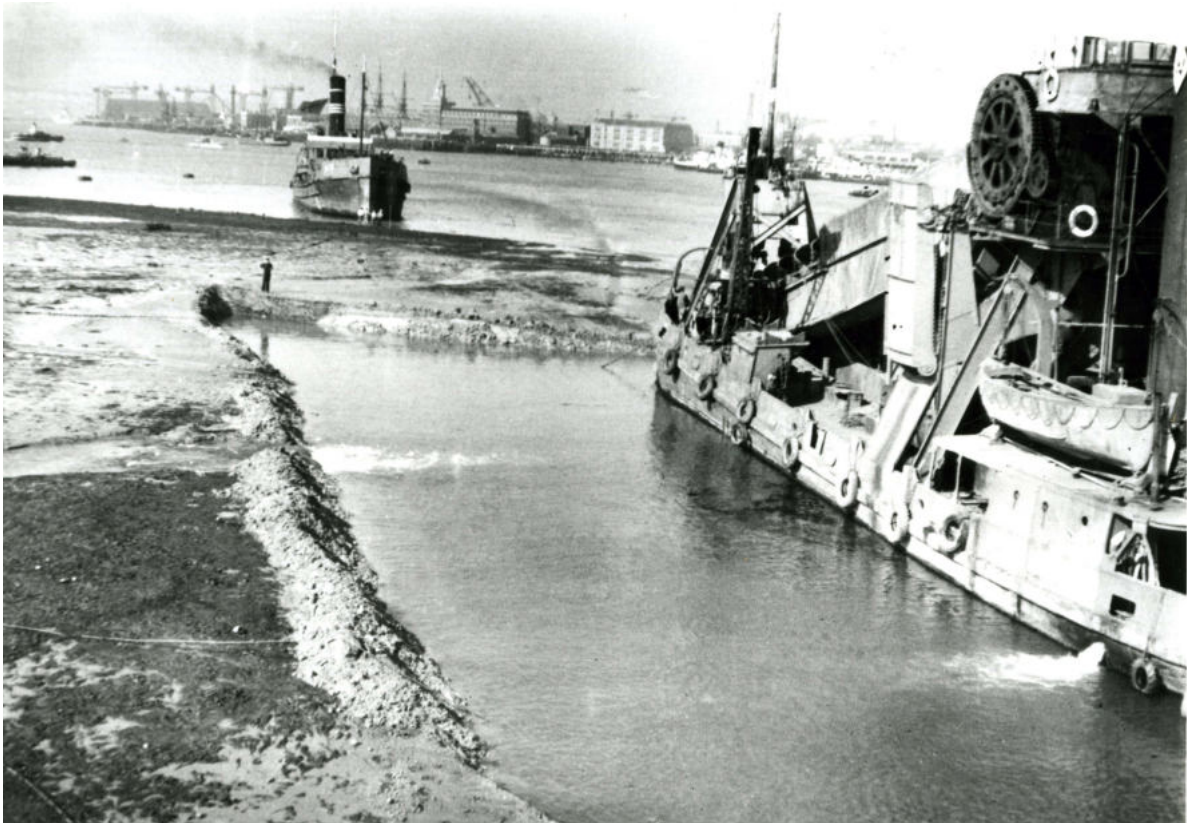
Figure 11 Conceivably the original ‘submarine’ dredge in which case the date is 1904. Note the man in the middle ground standing on the mud. MoD.
