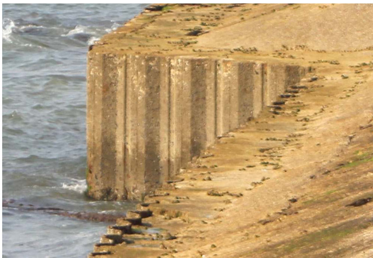
Figure 50 Aug 2020. Piles, last noted in place in photograph dated 2014, are now missing completely. Piles and concrete backing are parting company in the foreground. CHD.
