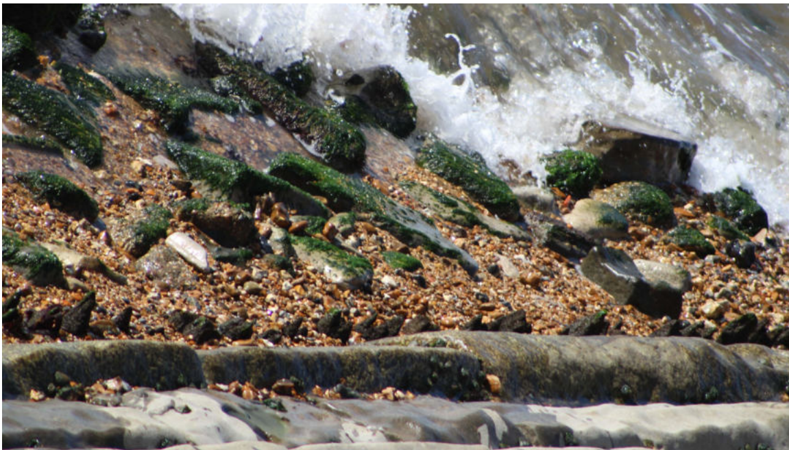
Figure 42 2019. Looking down from the top of the wall, close to the harbour entrance. For the first time in living memory, the remains of the piles, used when forming this part of the wall, are exposed. CHD.
