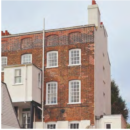
The rear of No. 1 showing the ablution block supported by steel columns.
