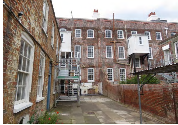
The rear of No. 1 showing the ablution block supported by steel columns.
