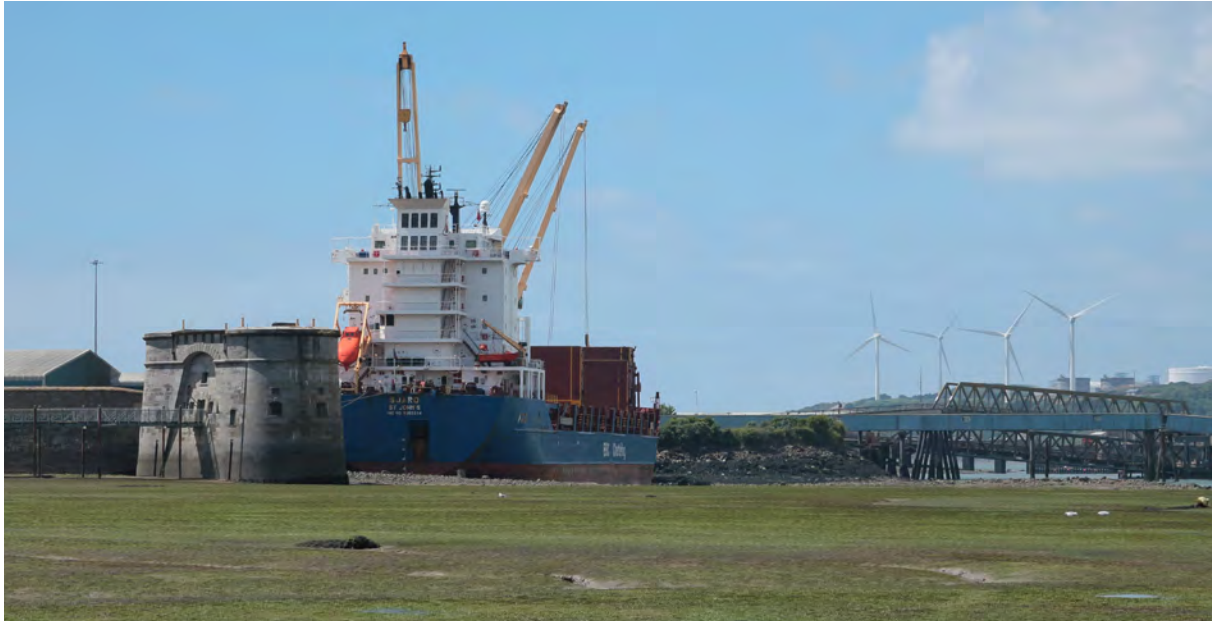
Northeast Martello Tower (1851), Pembroke Dock. Courtesy Rita Singer
