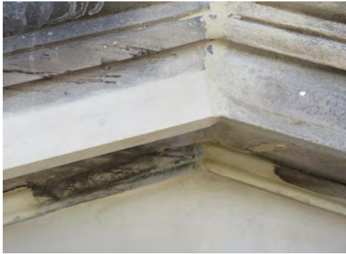
Sheerness Church: blending old and new sandstone in the entrance portico (above) and in the clocktower (right). (Ann Coats)
