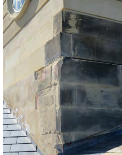
Sheerness Church: blending old and new sandstone in the entrance portico (above) and in the clocktower (right). (Ann Coats)
