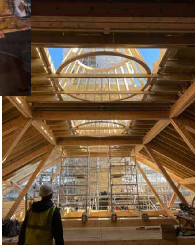
Right: The new roof framing and skylights looking towards the tower. February 2022. (Hugh Broughton Architects)
