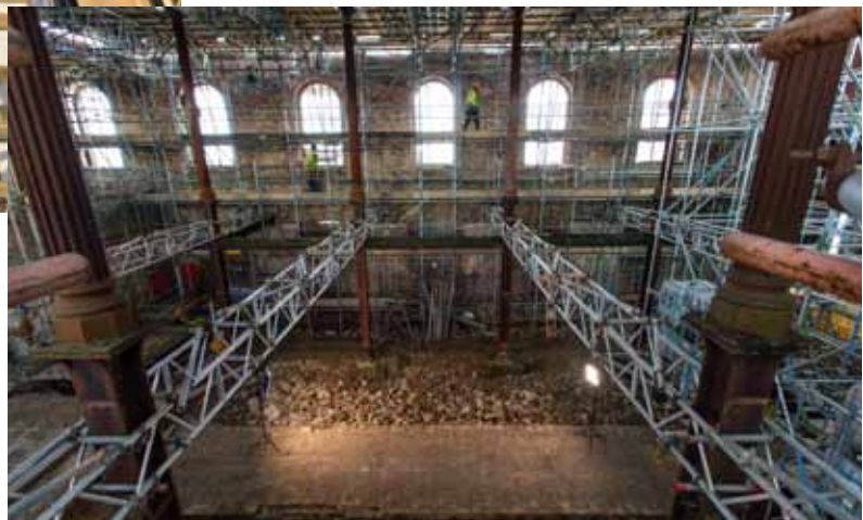
Right: Internal structural scaffolding framework. February 2021. (Toby Roney)
